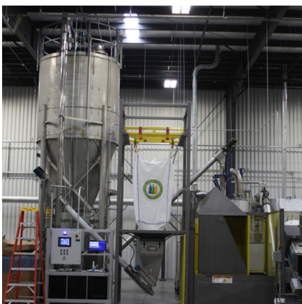
Bulk Bag Unloader, Flexible Screw Conveyor and Aero Mechanical Conveyor
