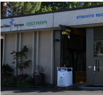
Clean Water Services' Nutrient Recovery Facility
