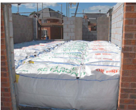
Typical use of a Soft Landing System in the Construction Industry
