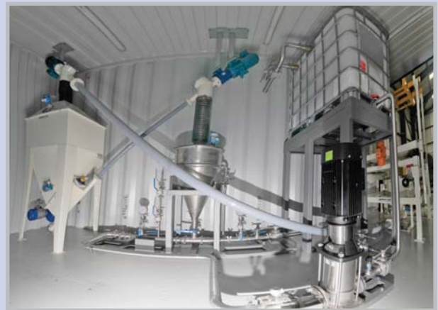
Water treatment system inside an ISO container
